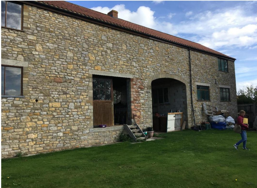
Fig 3. – Looking east – rear of the buildings to be converted
