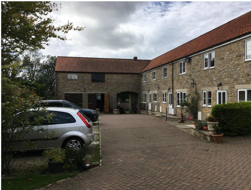
Fig 2. – Looking west towards the redundant outbuilding. Existing properties to right
